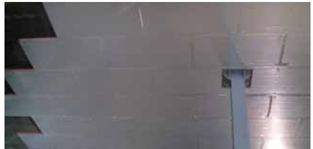
Figure 6 Board joints squared
